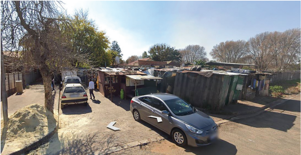
Figure 9. An illegal shack settlement on a suburban road, Concession Street in Jeppestown, north of the railway line. Source: Google Earth Street View, 2022. https://earth.google.com/web/search/Jeppestown+Johannesburg (accessed 15 August 2023).
