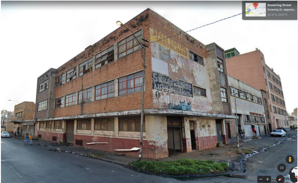
Figure 10. Gloomy 'monster' building. This factory building on the corner of Browning and Wolhuter Streets, Jeppetown, is visibly damp, with vegetation growing out of the brickwork. An open side door hints that people may be living in this horrible place.
